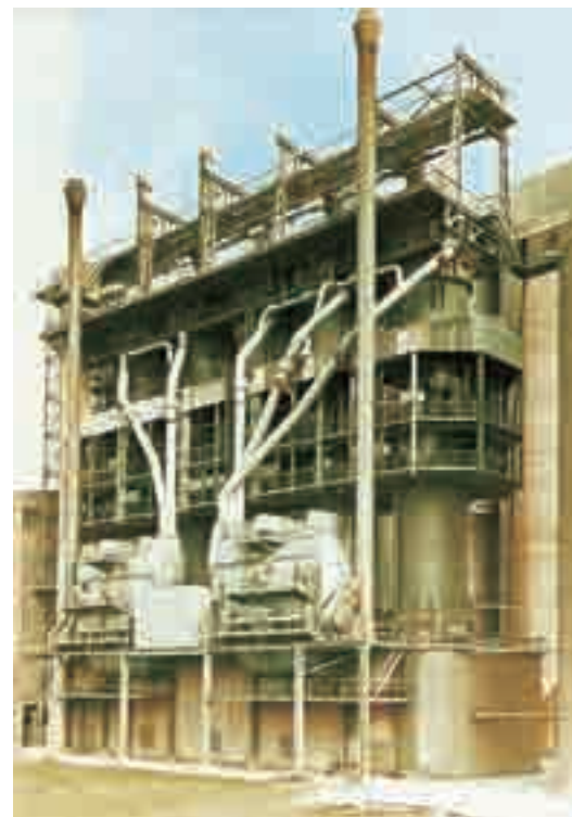
Shaft furnaces in which slaked lime is manufactured from limestone (photo: Dyckerhoff AG, Lengerich plant)
